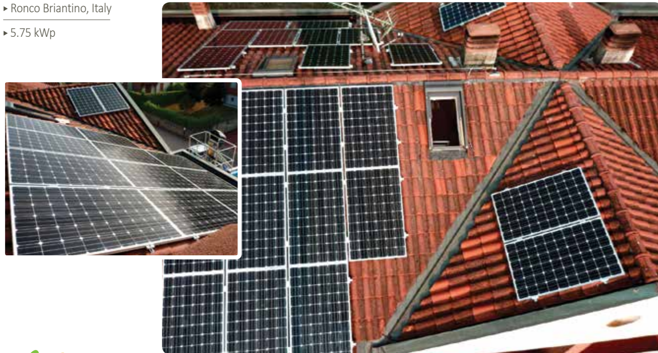
The SolarEdge DC optimized inverter system enabled five additional panels to be installed and only required one 23-panel string - despite the roof having asymmetrical and opposite-facing facets.
