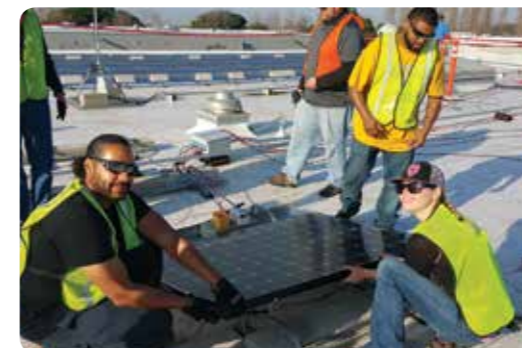
Teamwork to take this roof solar
