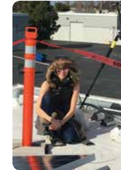
Staying cool with rooftop PV
