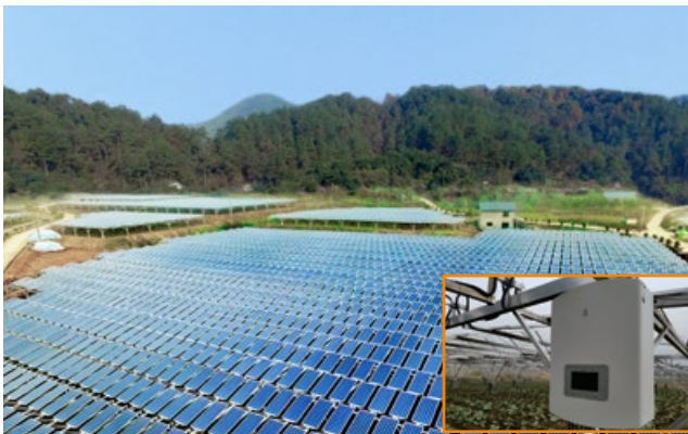
Zhejiang Dajie Agricultural-photovoltaic hybrid PV plant 3MW
