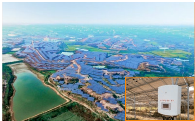
Zhejiang Longyou Agricultural-photovoltaic hybrid PV plant 25MW
