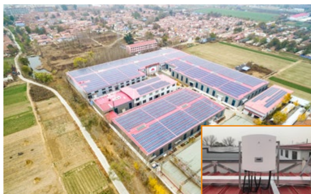
Shandong YUELONG 3.5MW
