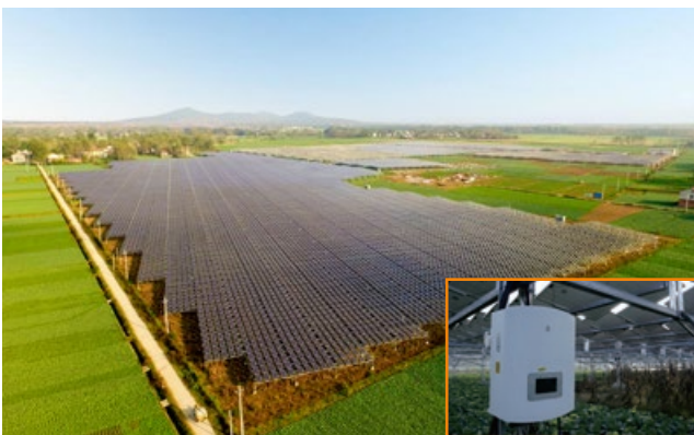
Hubei Guanyin Agricultural-photovoltaic hybrid PV plant 20MW
