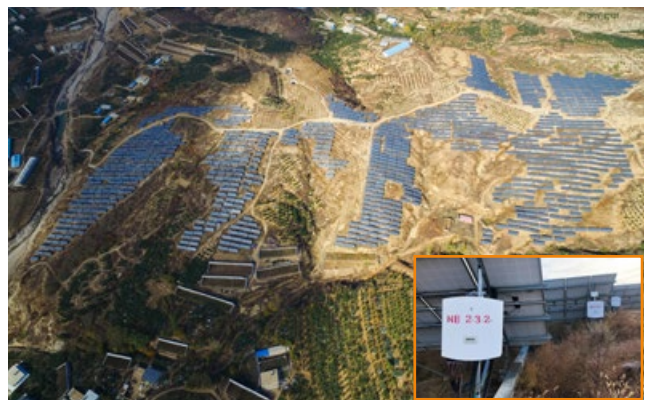
Liaoning Jiuzhai Gaizhou PV plant 20MW
