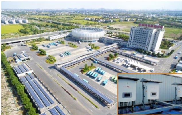
Zhejiang PINGHU Bus Station 472kW
