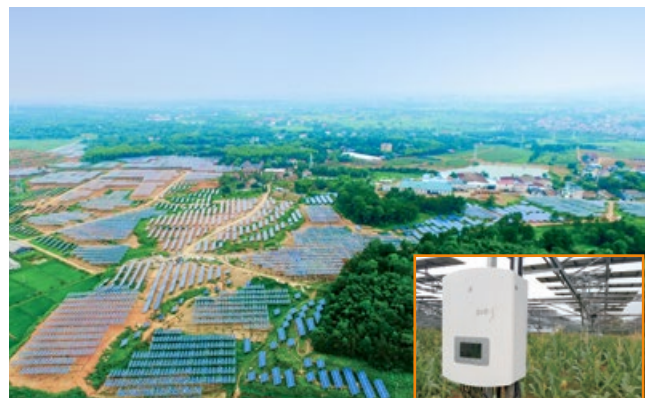
Quzhou Qinghu Agricultural-photovoltaic hybrid PV plant 20MW
