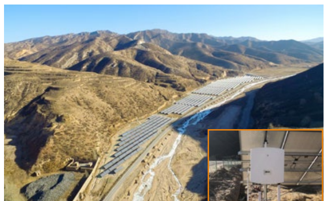
Shanxi Yizhou Jingle poverty alleviation PV Plant 36.3MW
