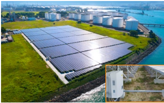
JTC Solar Farm, Singapore 5MW
